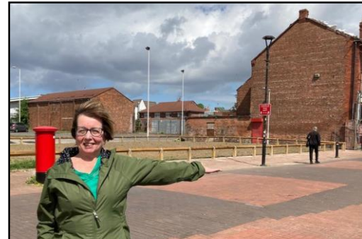
Ruth Molyneux before and after the site preparation for new homes in New Ferry.
